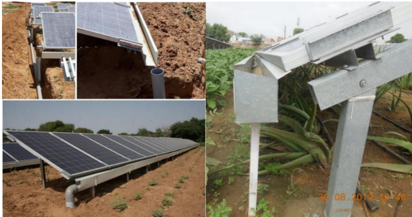
Figure 41: Ground mounted agrivoltaic system with integrated rain gutter for collecting rain-water. 156
