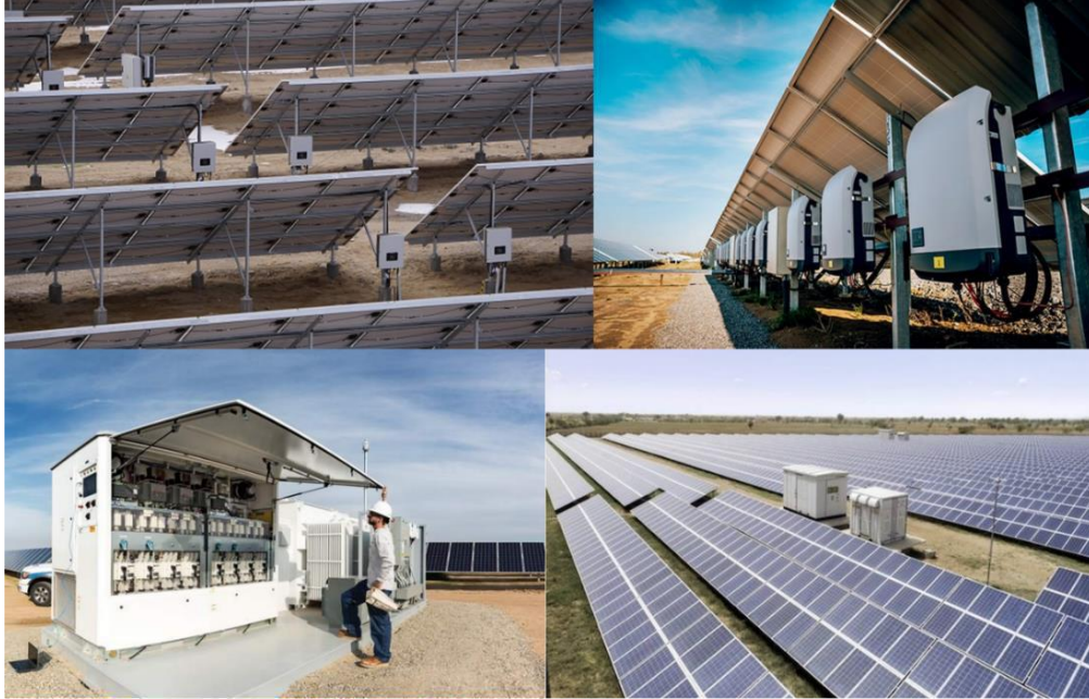
Figure 21: Comparison of String (top) & Central inverter (bottom).
