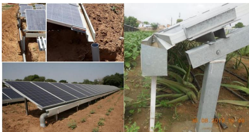
Figure 17: Ground-mounted agrivoltaic system with integrated rain gutter. 44
