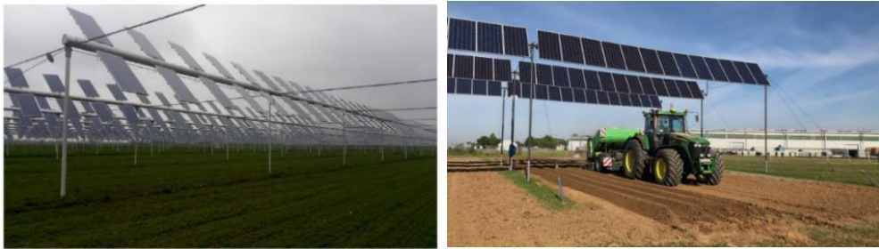
Figure 19: Tensile structures of (a) the tracked agrivoltaic system (Agostini et al., 2021) and (b) a static overhead system © Krinner Carport
