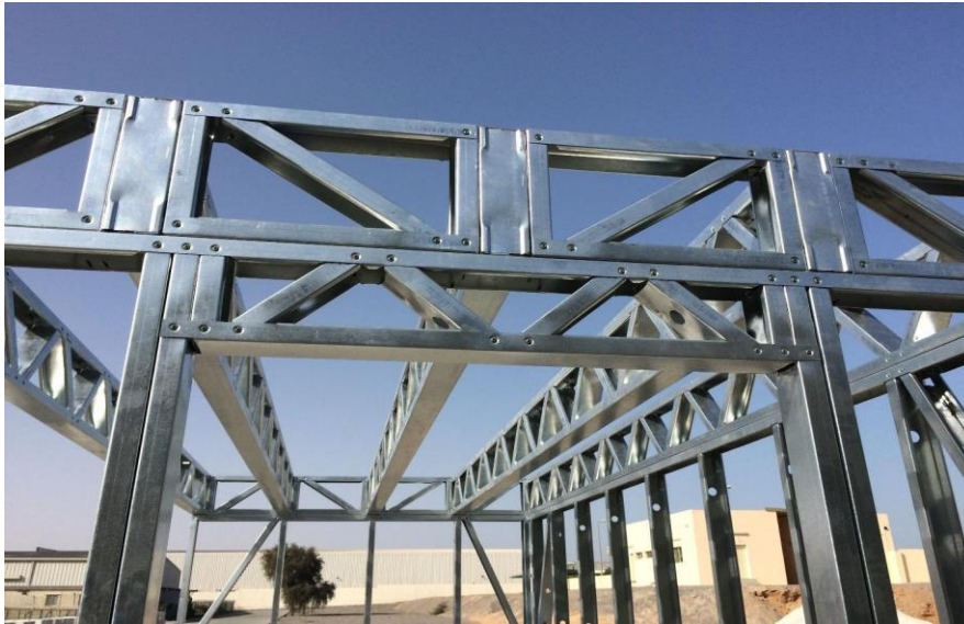
Figure 13: Floor, roof truss, beam arrangement
