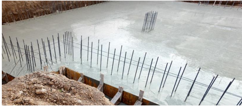
Figure 2: Raft foundation Construction (Kolos Cement Ltd, 2019)
