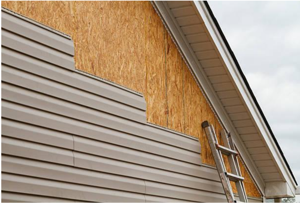
Figure 9: Vinyl sliding on OSB board
